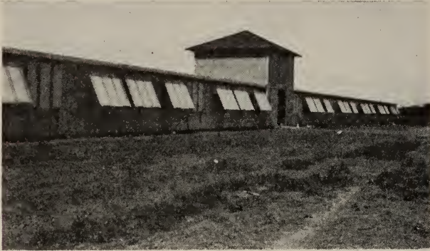
Fig. 10.—The three-purpose curtain. Some are shown held out at bottom to shade open front without restricting ventilation; others are closed down over front openings as they would be in stormy weather. In the frontispiece, these curtains are also shown with inner panels open to admit direct sunlight into house. Details of the construction of this curtain shown in figure 11.
